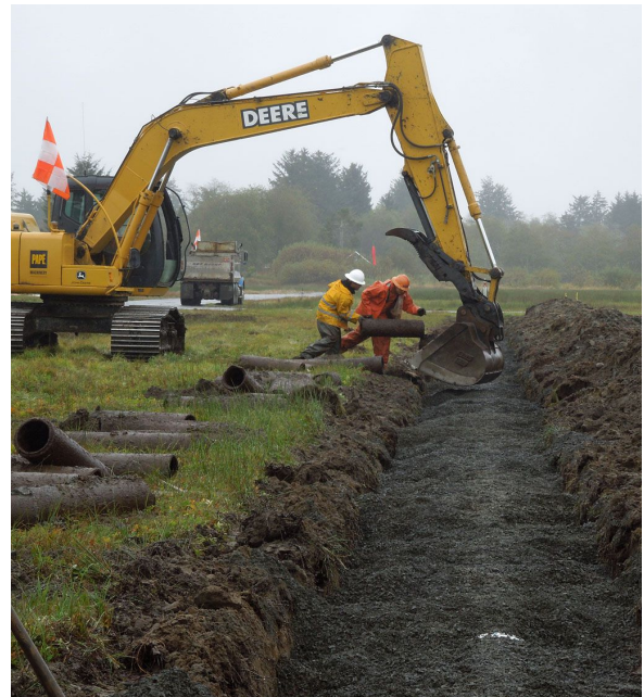
Local contractors replacing failed drainage pipes, fall 2011.
